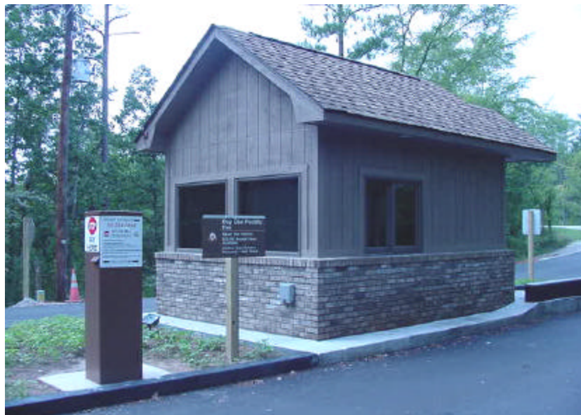
Photo I-18. Honor vault at entrance station, Example 2. J. Strom Thurmond Lake, SC. This style of vault incorporates associated signage on the unit itself (Para. 4.10.1)
