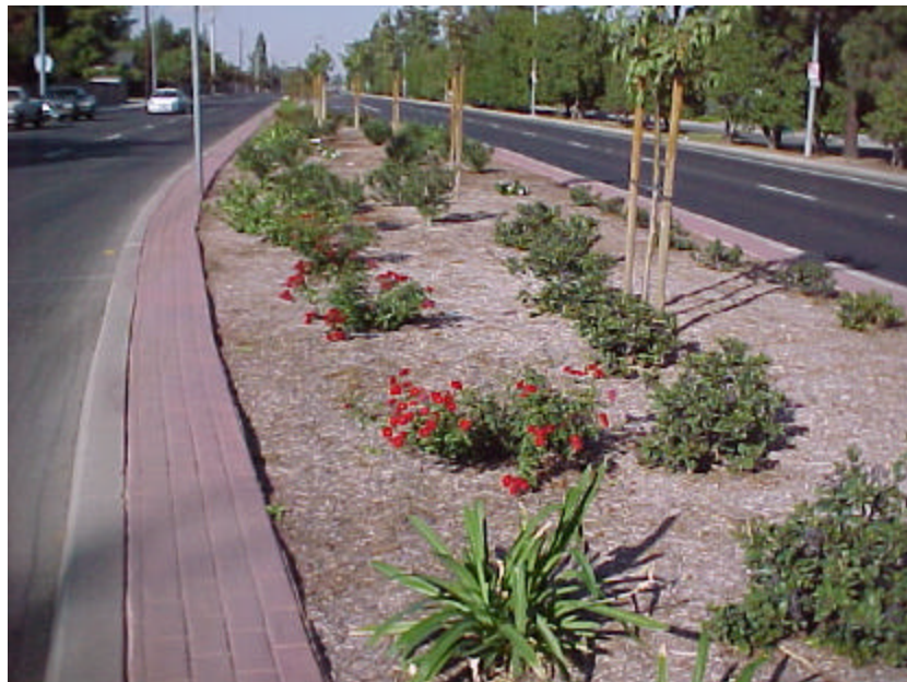
Photo I-5. Clovis, CA. Landscape features, Example 3. Low maintenance isolated area in the median eliminates mowing requirements. Flowers and trees (all indigenous, drought tolerant) established with weed barrier fabric and mulched to prevent weed growth. Irrigation hidden in vegetation. Edging set flush with ground level. Paras. 2.7.2 and 2.7.3
