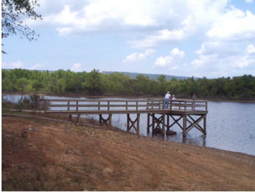
Photo N-15. Fishing pier, Example 3. Nimrod Lake, AR. This fixed fishing pier is not located in a park, but at the end of a gravel lake access road on the bank of an underwater stream. Local senior anglers chose the location because of the good fishing (Tables 5.9 and 5.10)
