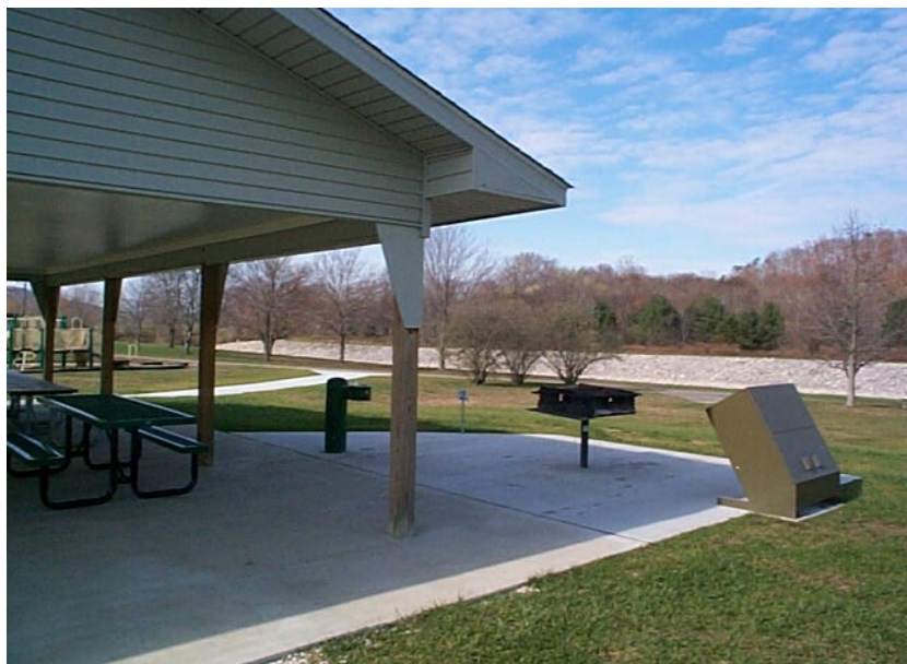
Photo P-8. Picnic shelter features and amenities, View 2. Cave Run Lake, KY. Shelter has low-maintenance vinyl siding at gable ends. Extended concrete apron accommodates UA grill, UA drinking fountain, and garbage containers with UA (side opening) doors (Table 3.2)
