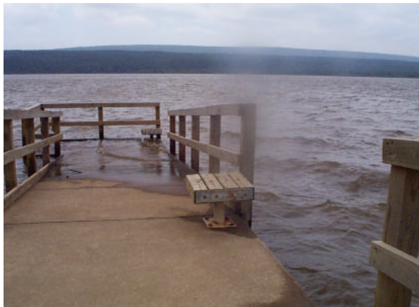
Photo N-12. UA boat loading platform, Example 2. Carter Cove Park, Nimrod Lake, AR. This is a custom design with a series of ramps and landings that are 1.5 ft apart in elevation. When one landing becomes unusable due to rising water, the next one is usable (Table 5.8)
