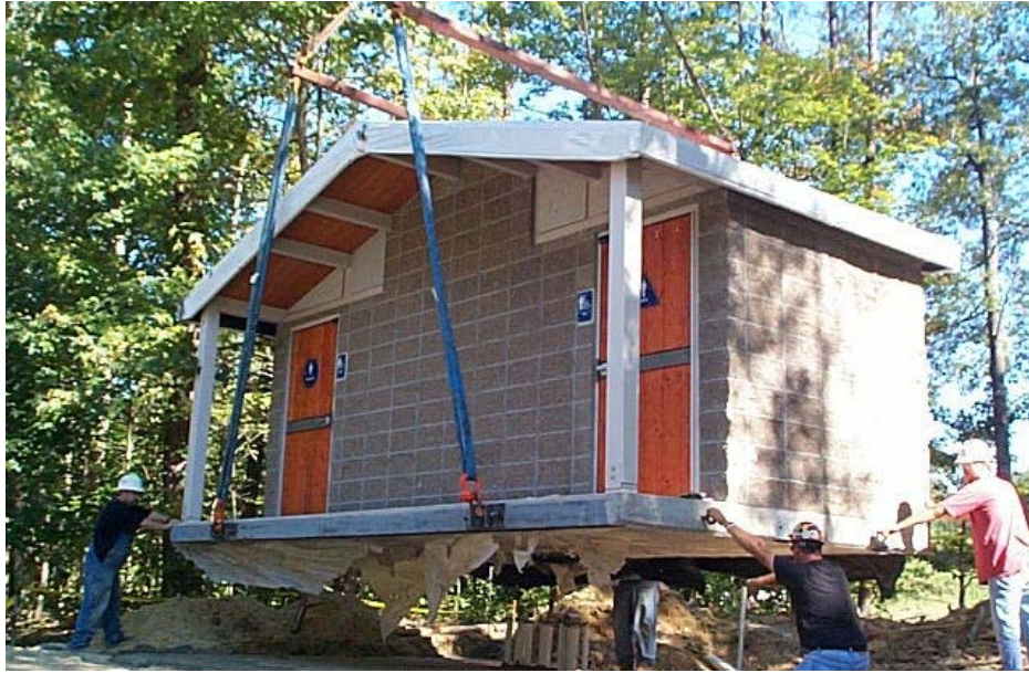
Photo K-3. Prefab restroom building. High Bank Recreation Area, Cave Run Lake, KY. Installation of a prefab building shows some advantages of using commercially available units (para. 1.21)
