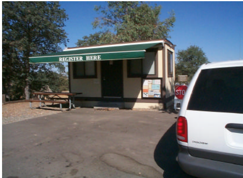
Photo J-10. Customer service window overhang, Example 2. Cordoniz Recreation Area, Eastman Lake, CA. An automated retractable awning is installed at this walk-up outside customer service window (Table 3.1)
