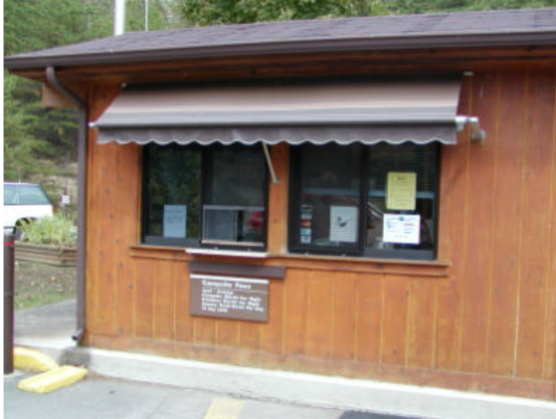
Photo J-9. Customer service window overhang, Example 1. Littcarr Campground, Carr Creek Lake, KY. A retractable RV awning installed to provide customers with protection from the elements while they conduct business at this drive-up outside customer service window (Table 3.1)
