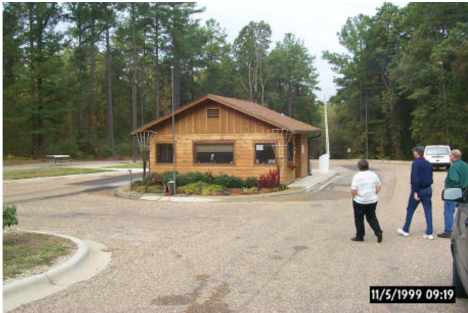
Photo J-2. Entrance station features. Brushy Creek Park, Lake O' the Pines, TX. Note building design and landscaping are in keeping with the theme of the area, and low-maintenance building exterior. Optional dual lanes and recommended turnaround incorporated for customer convenience (Table 3.1)
