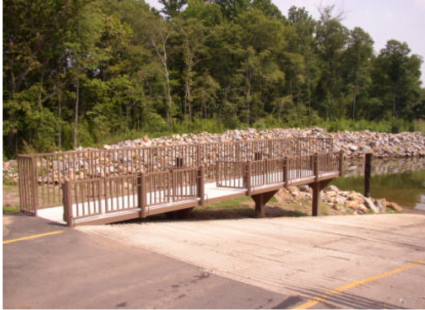
Photo N-11. UA boat loading platform, Example 1. Spadra Park, Lake Dardanelle, AR. Constructed by the Arkansas Game and Fish Commission, this design provides several gates along the length of the dock and stable support as customer enters boat (Table 5.8)
