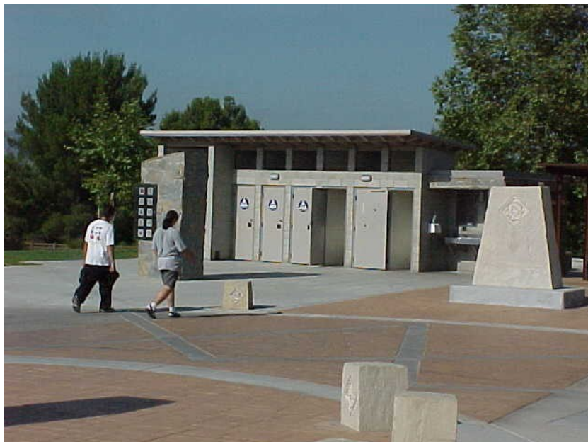
Photo K-2. Unisex restroom with family room. Lake Balboa, Los Angeles Department of Recreation and Parks, Los Angeles District. Example of a unisex restroom building (Paras. 3.5.1 and 3.5.2)
