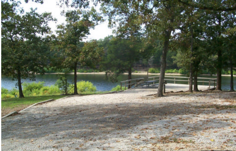
Photo M-7. Camping spur follows terrain - Example 1. Pomme de Terre Lake, MO. (Table 5.1). This photo also demonstrates hardened living area located on the passenger side, timber border, provision of room for RV slideouts, and required site amenities (Table 5.4)
