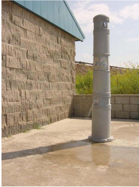
Photo K-13. Change house outdoor shower. Sandy Park, Canton Lake, OK. Outside shower provides for sand removal. Note multilevel shower heads (Table 3.9)
