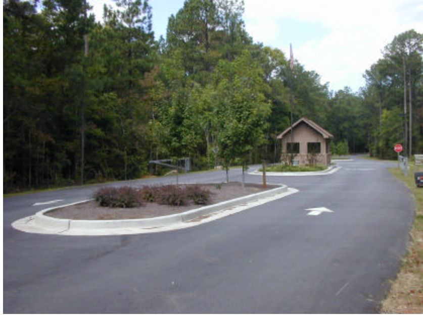
Photo J-1. Entrance station island. Winfield Campground, J. Strom Thurmond Lake, GA. Note recommended center of roadway entrance station location, turnaround incorporated into entrance station approach, and roadway markings to direct traffic flow (Table 3.1)
