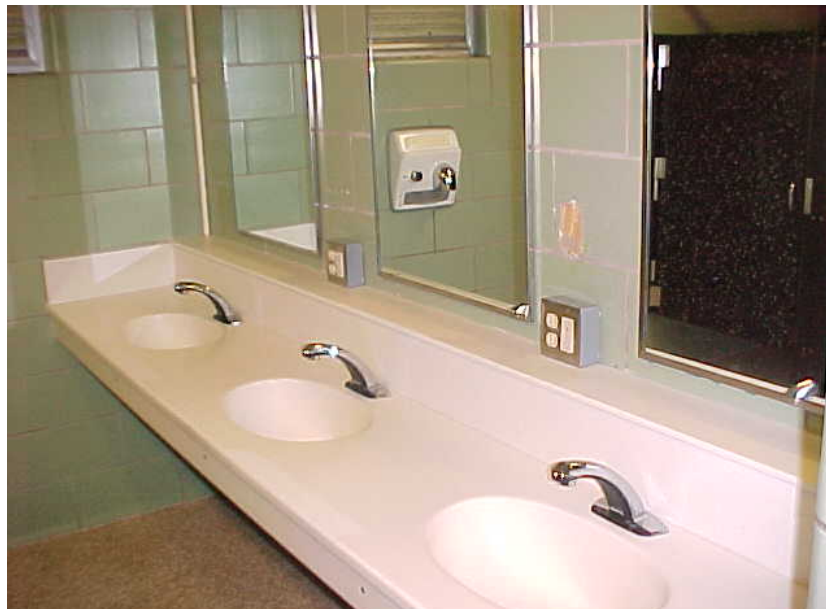
Photo K-6. Sinks incorporated into countertops. North Fork Campground, Rough River Lake, KY. Customers like the additional counter space. Also note that a GFCI protected outlet is provided for every two sinks, and motion-activated faucets have been included (Tables 3.4 and 3.5)
