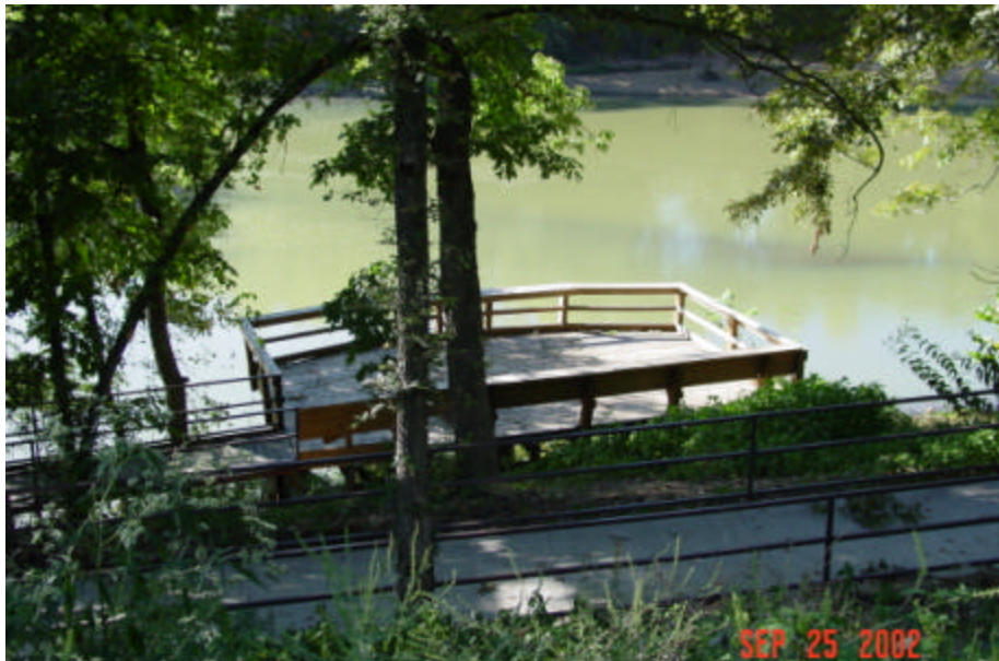
Photo N-16. Fishing pier, Example 4. Trout Stream Access Point, Tenkiller Ferry Lake, OK. This UA pier is a fixed design. Note the access ramp in foreground (Tables 5.9 and 5.10)
