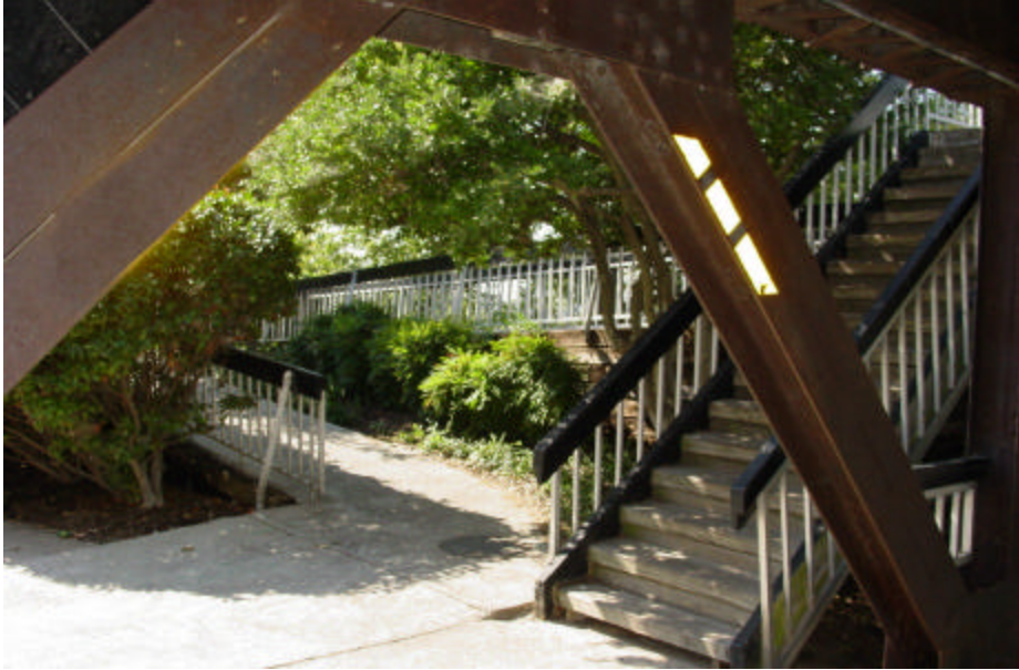
Photo I-1. UA ramp combined with steps. Tulsa River Parks, OK. Along with a UA access ramp, limited use of stepped designs may be incorporated when necessary to fit within the existing topography, facilities, and pathways (Para. 2.10)
