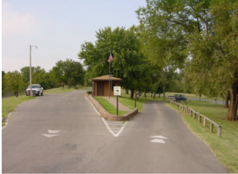
Photo J-3. Dual lanes, Example 1. Canadian Park, Canton Lake, OK. This is the view exiting the park. Note the dual entrance lanes, arrows on pavement designating traffic flow (Table 3.1)
