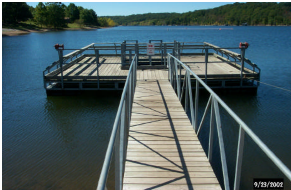
Photo N-14. Fishing pier, Example 2. Prairie Creek Recreation Area, Beaver Lake, AR. This UA pier includes a fishing well, and resulted from a partnering effort between the Corps, the Arkansas Game & Fish Commission, and local bass clubs (Tables 5.9 and 5.10)
