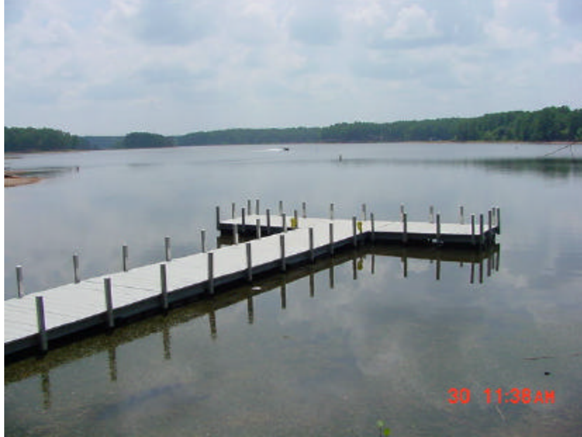
Photo N-7. Courtesy dock, Example 3. Amity Boat Ramp, Thurmond Lake, GA. Floating design, recycled plastic decking (Table 5.9)
