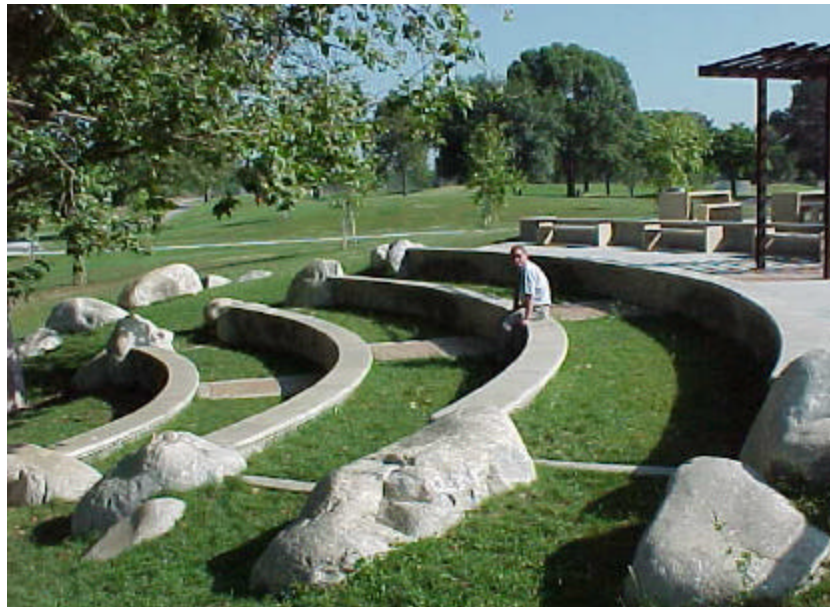
Photo M-16. Low-maintenance amphitheater. City of Los Angeles outgrant, Lake Balboa, Los Angeles District. Amphitheater is constructed of low-maintenance materials that are indigenous to the site. This is an example of a sustainable design. Note that top section is UA (Para. 5.4.8.1)
