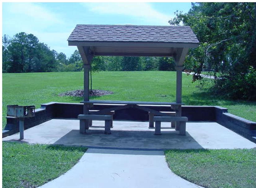
Photo P-12. UA covered table. West Dam Day Use Area, J. Strom Thurmond Lake, GA. Shade structure constructed to provide shade for table (Table 5.13). Note UA features: concrete walk and pad, and split bench design that allows wheelchairs or strollers to pull up to the table (Para. 5.2.1)
