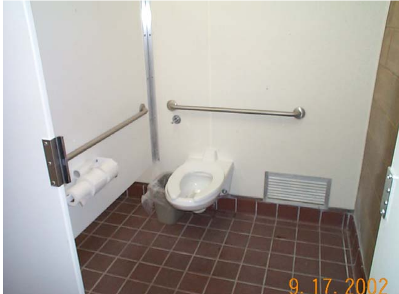
Photo K-11. Interior color contrast. Robinson Point Park, Norfolk Lake, AR. Note the required floor and wall contrast at base (Table 3.7). Also note that this is a UA stall
