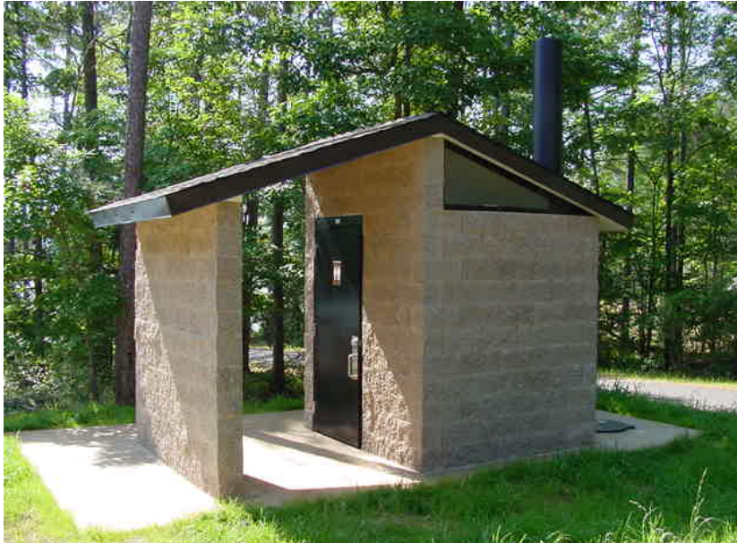
Photo K-1. Unisex vault restroom. Dordon Creek Boat Ramp, J. Strom Thurmond Lake. Example of the minimum restroom facility that may be provided (Paras. 3.5.1 and 3.5.2)
