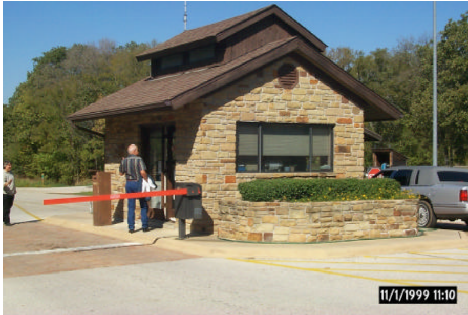
Photo J-11. Automatic gate. Hickory Creek Park, Lewisville Lake, TX. Automatic gate can be operated from inside the entrance station and allows after-hours departures
