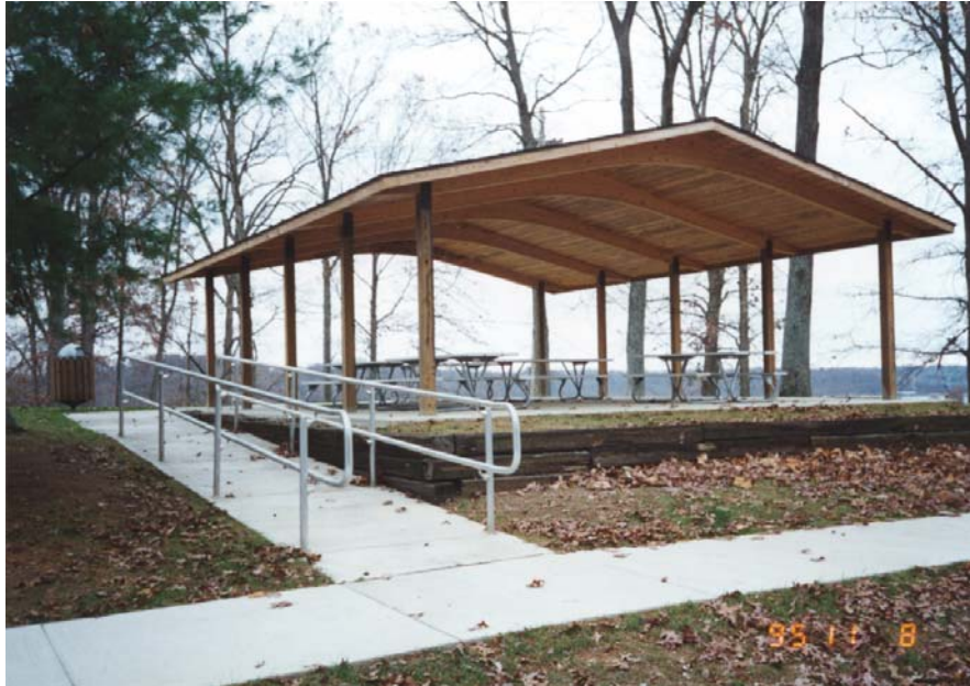
Photo P-3. Picnic shelter roof trusses. Overlook Area, Monroe Lake, IN. Note that roof trusses do not allow birds to roost or build nests (Table 3.2). This shelter constructed from a prefab kit. Also note railings incorporated on sidewalk for UA
