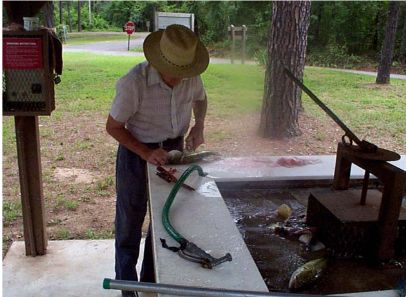
Photo L-3. Customer using fish-cleaning station. Carter Cove Park, Nimrod Lake, AR. This station includes two water hoses with spray nozzles, a 2-hp grinder with timed start/stop switch and custom cover (fish remains go into septic tank and leach field), GFCI receptacles, and night lighting (Table 3.10)
