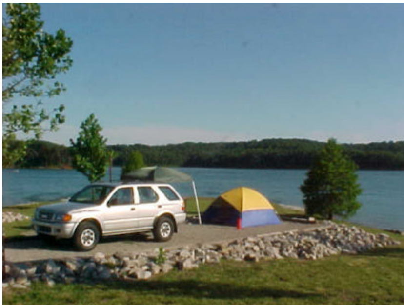
Photo M-4. Hardened living area. Moutardier Campground, Nolin River Lake, KY. Fine crushed stone surface provided (Para. 5.3.3.1)
