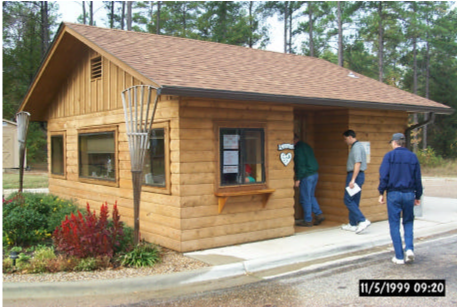
Photo J-7. Customer service window and walk-in area. Brushy Creek Park, Lake O' the Pines, TX. Customers are shown entering walk-in area of entrance station. Note that an outside service window is also provided (Table 3.1)
