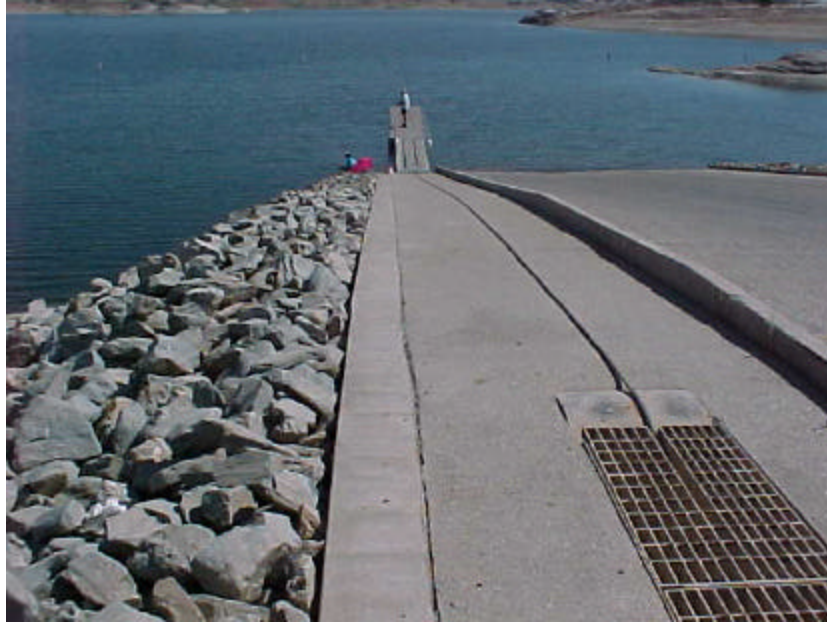
Photo N-3. Wave erosion protection. Hensley Lake. Riprap or quarry run rock is the minimum protective edging provided to protect boat launching ramps from erosion due to wave action (Table 5.8). Also note guide cable anchoring system (Para. 5.4.2)
