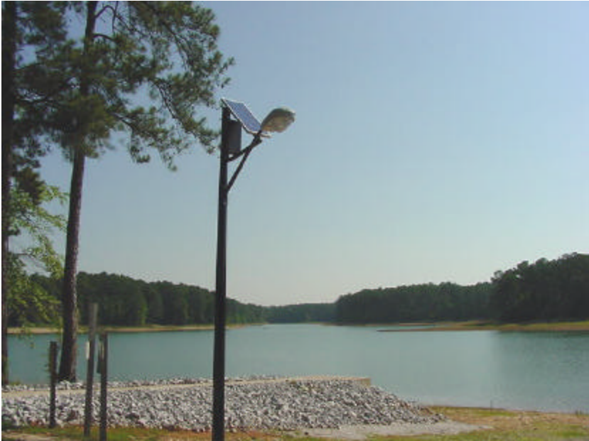
Photo I-2. Solar-powered lighting. Dordon Creek Boat Ramp, J. Strom Thurmond, SC. Solar is an option to provide lighting at areas where electrical service is not available (Table 2.7)
