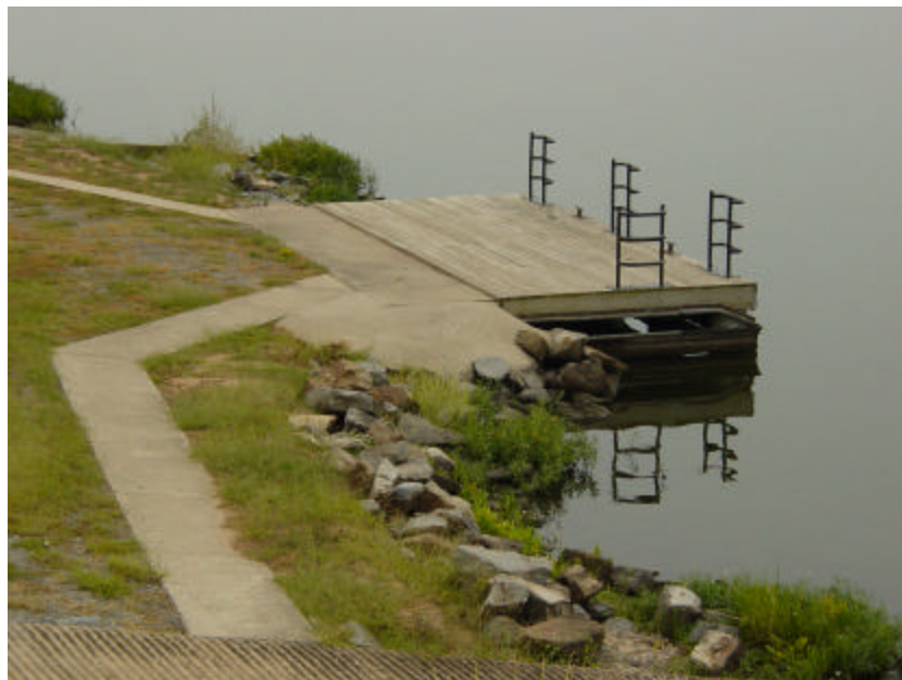
Photo N-8. Courtesy dock, Example 4. Ste. Marie Park, Lower Arkansas River. This fixed dock features handrail/ladder combinations for assistance in entering boats (Table 5.9)
