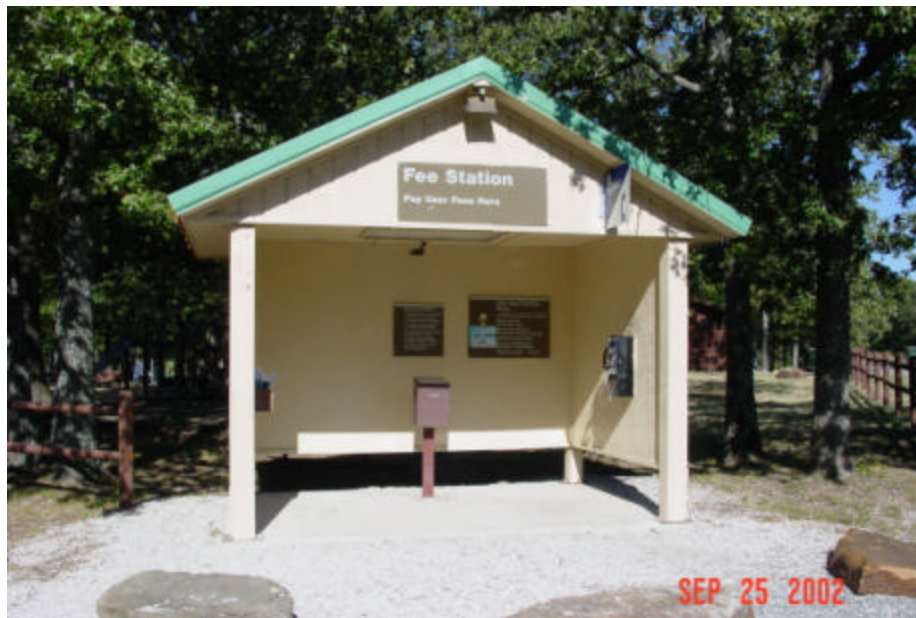
Photo I-16. Honor vault - day use area, Example 2. Snake Creek Recreation Area, Tenkiller Ferry Lake, OK. This example includes a shelter for users that incorporates lighting and a pay phone (Para. 4.10, 4.10.1)
