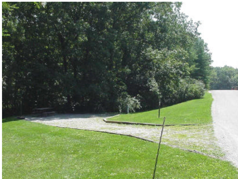
Photo M-8. Camping spur follows terrain - Example 2. Note how cut and fill are avoided by building this back-in site on the contour (Table 5.1)
