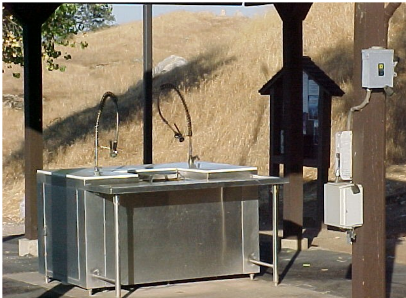
Photo L-2. Interior view of fish-cleaning station. Hensley Lake, CA. Note that this fish-cleaning station has a UA maneuver area, is sited on a concrete pad, and that two water hydrants are provided (Table 3.10). UA utility sink should be a feature of new units
