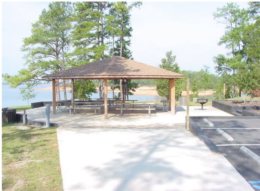
Photo P-2. Picnic shelter concrete pad. Clarks Hill Park, Hannah Point Shelter, J. Strom Thurmond Lake, SC. Note that concrete pad extends beyond the edge of the support posts for UA, and is sloped to drain away from the shelter (Table 3.2)
