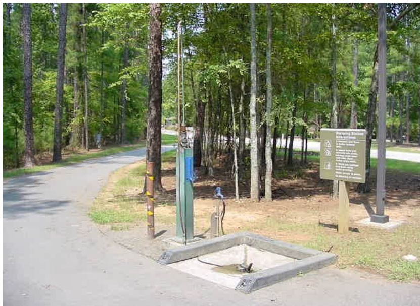
Photo L-4. Sewage dump station. Petersburg Campground, J. Strom Thurmond Lake, GA. This view shows wash down and signage. The potable water spigot is outside of photo (Table 3.11)
