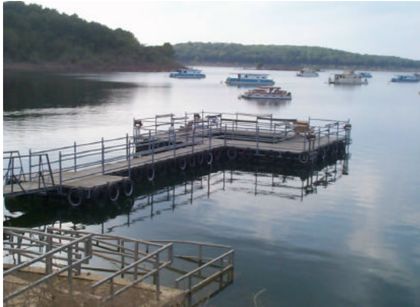
Photo N-13. Fishing pier, Example 1. Bull Shoals Park, Bull Shoals Lake, AR. This design includes a fishing well in the center of the floating pier (Tables 5.9 and 5.10)
