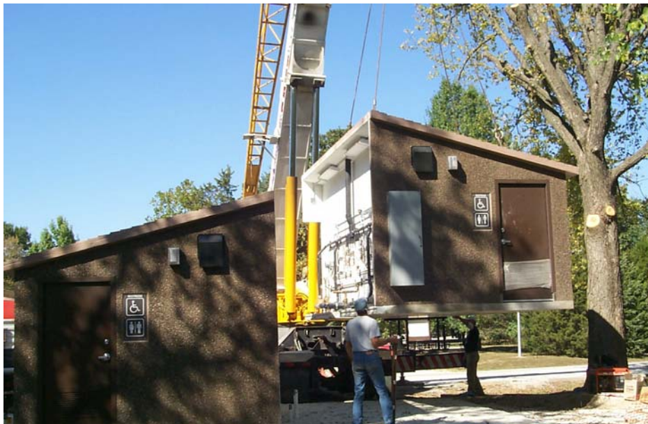
Photo K-4. Prefab unisex shower house. Nemo Park, Pomme de Terre Lake, MO. Installation of a prefab building shows some advantages of using commercially available units (Paras. 1.21 and 3.5.2)
