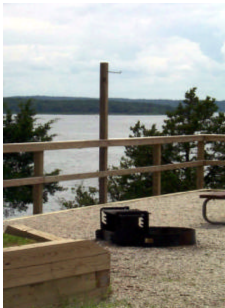
Photo I-14. Lantern hanger incorporated into railing. Damsite Park, Pomme de Terre Lake, MO. Lantern hanger placement and construction blends with campsite (Table 4.3)
