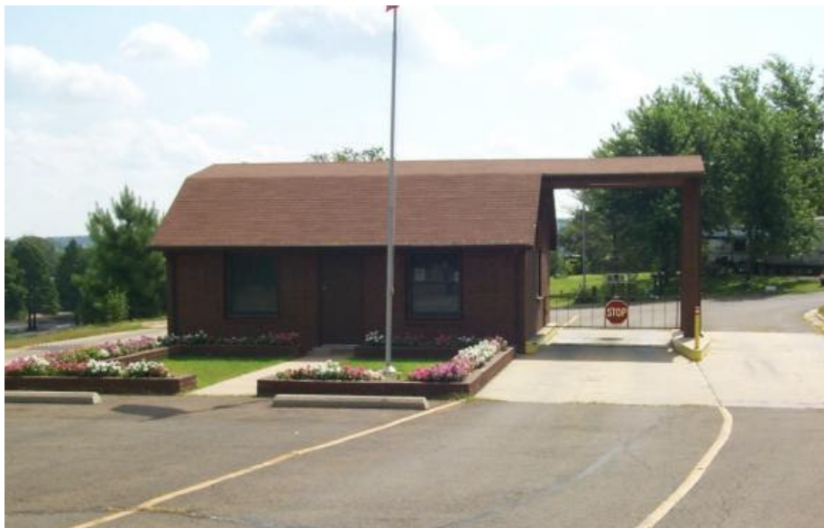
Photo J-4. Dual lanes, Example 2. Taylor Ferry Park, Ft. Gibson Lake, OK. Note dual entrance lanes, traffic control gate, customer parking in front of building so pedestrians do not cross traffic lanes (Table 3.1)
