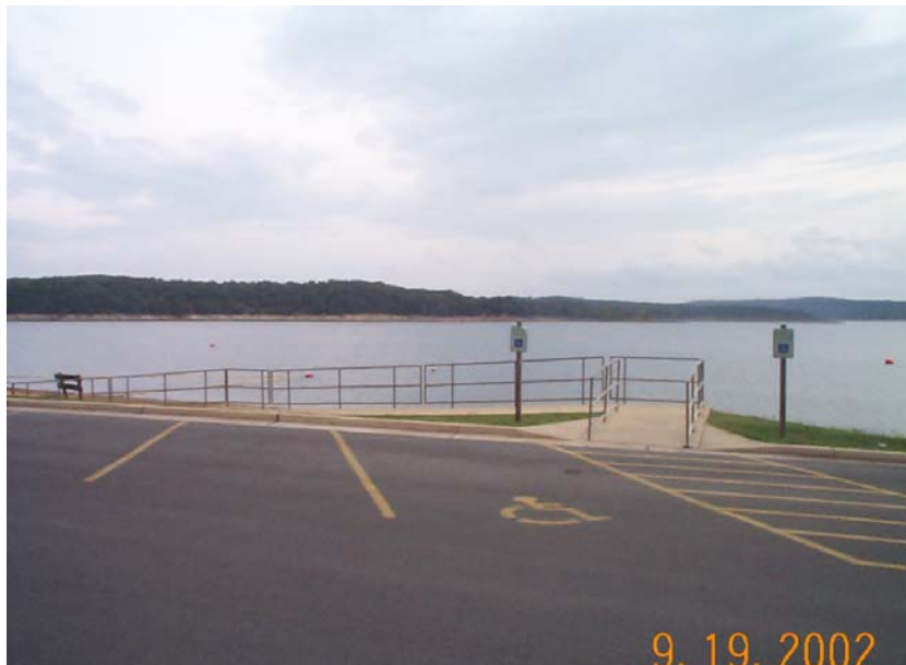
Photo O-2. UA ramp to swimming area. Cranfield Park, Norfolk Lake, AR. A concrete ramp from the parking lot to the swimming area enables wheelchair users to access the water (Para. 5.2.1)
